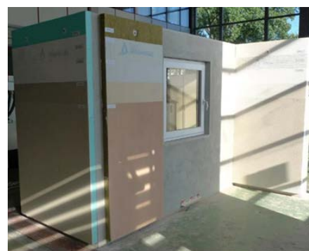
On the left: Training of trainees at CICCOPN, in Maia; on the right: practical training model of a wall with different types of ETICS applied.
